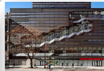
The New School University, NYC 40,000 GPD in-building onsite water treatment & reuse for flushwater, cooling, irrigation & laundry.
