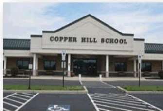
Copper Hill Elementary School, East Amwell, NJ 1 st public school water reuse system.
